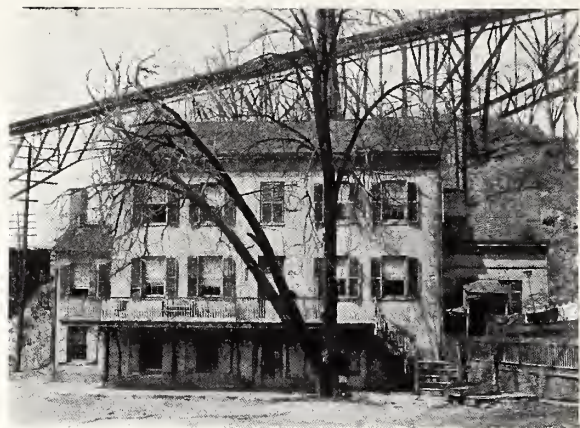
Reynolds House, built by James Reynolds near Upper Landing, (and ferry), about 1827.
